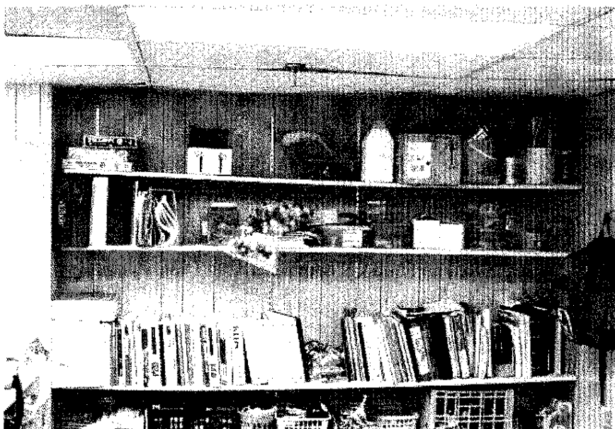
DAMAGE IS visible in the counselor's office in the basement of the elementary school.
